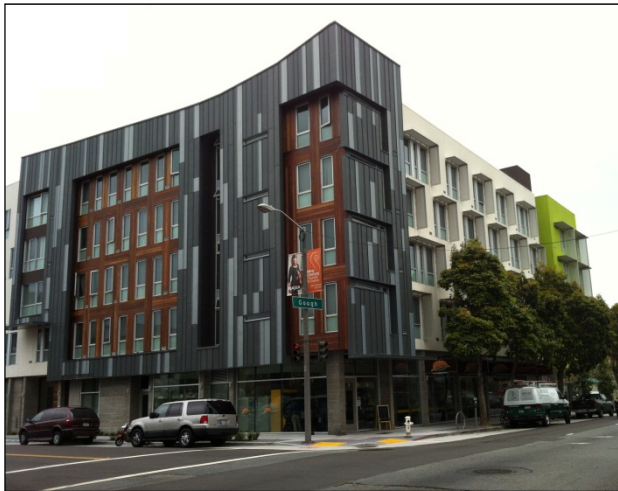
The new Richardson Apartments at Fell and Gough are operated by Community Housing Partnerships. Redeveloped in partnership with Mercy Housing California, the facility won recognition for its innovative design.
