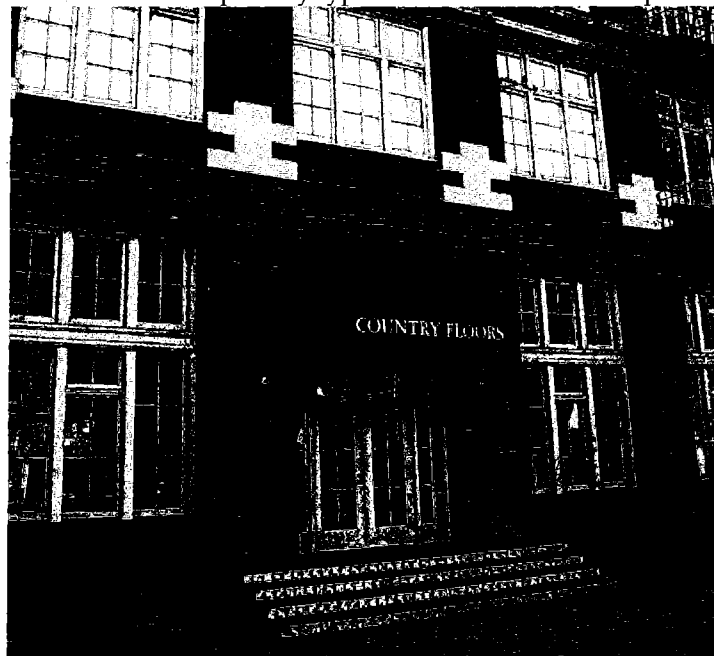
Detail: Contemporary exterior stair, northwest facade
