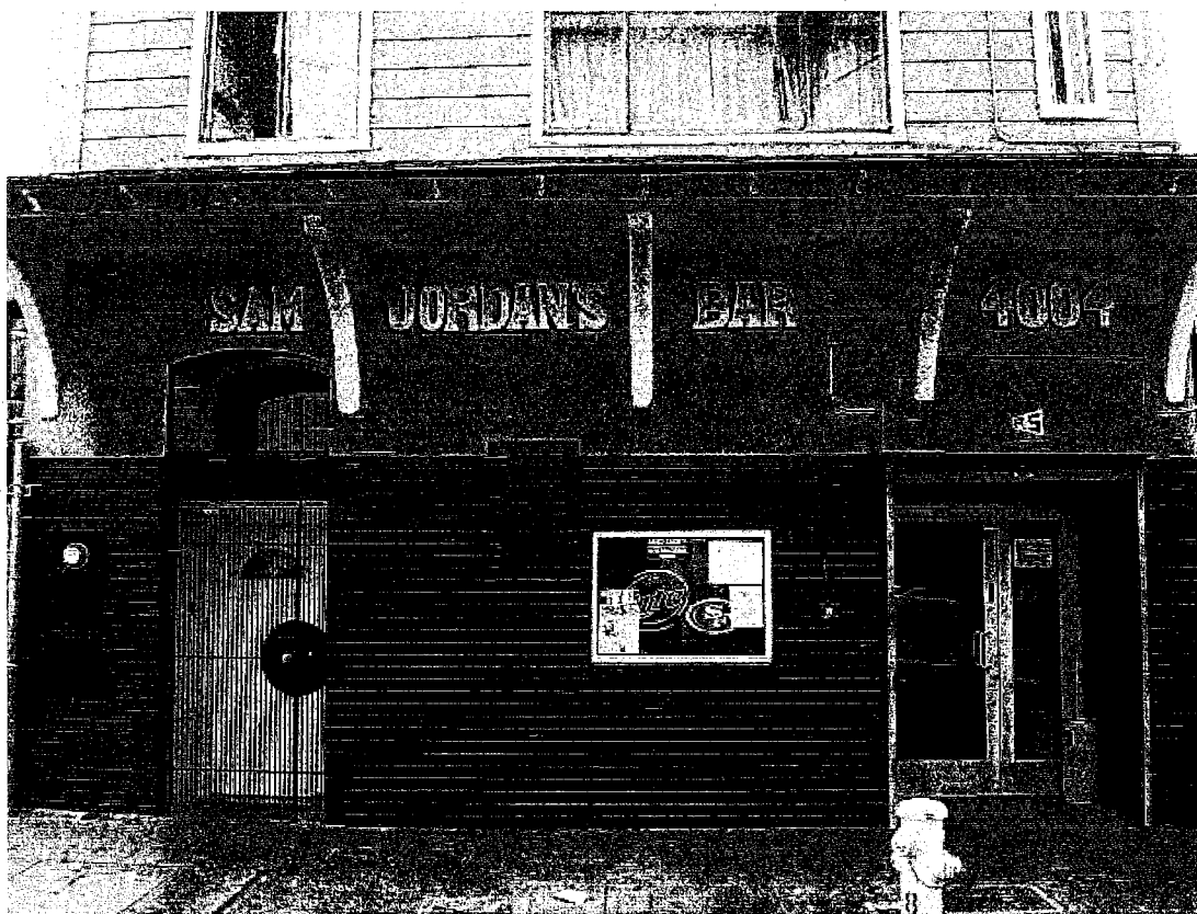
First story, primary facade.
