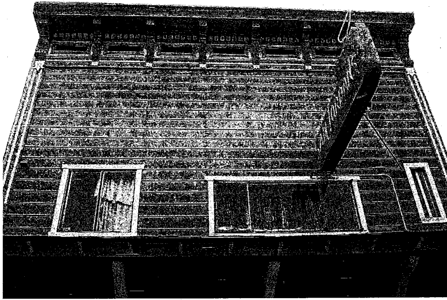
Second story, primary facade.
